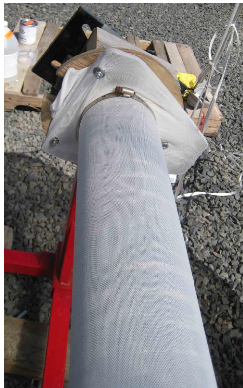
Photos 6 & 7. The mast ground down through most of the gelcoat to the glass, but not all the way through. The glass sock put on. This owner used a tube fabric from Giant Leap Rocketry: http://giantleaprocketry.com/products/components_composites.aspx .
