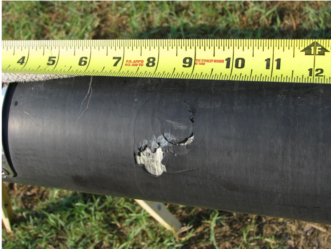
Photo 3. Impact damage on a Freedom 21 mast, showing gelcoat and underlying glass.
